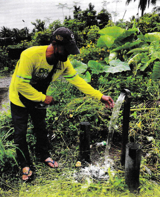
PrimeWater's Edmund Llapitan checking the residual chlorine at one of the blow-off points inside Executive Village last October 28.
