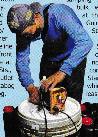
PrimeWater quality personnel Edmund J. Llapitan installing the hypochlorinator during the 'Oplan Linis Tubo' at BLISS, Apr. 25
